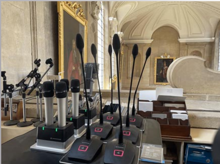
Page 22 - Sennheiser shows how to cope when installing audio in historic buildings.
